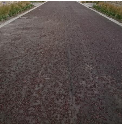
Stone Chip rolled into Tarmac Surface to act as shared surface.
